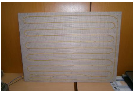
Figure 8 - Detail of installation of heating cable
