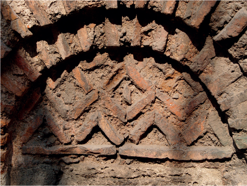
Figure 5: Brickwork patterns. Bottom zone of the apse, Saint John the Baptist, Constantinople. Photo by Jasmina S. Ćirić.
