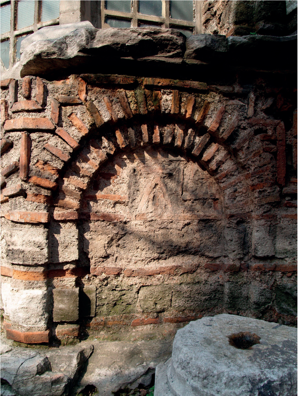
Figure 6: Triangle brick pattern. Bottom zone of the apse, Saint John the Baptist, Constantinople. Photo by Jasmina S. Ćirić.
