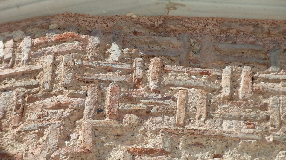
Figure 15: Brick pattern. Upper zone, apse, detail, Saint John the Baptist, Constantinople. Photo by Vladimir Božinović.
