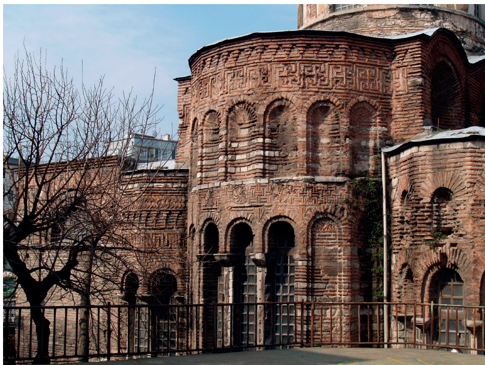
Figure 2: East façade from the North. Saint John the Baptist, Constantinople. Photo by Jasmina S. Ćirić.
