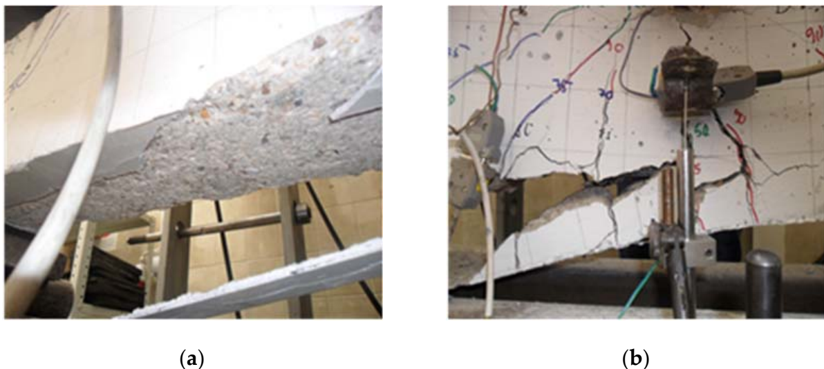
Figure 21. Beam B-EC: (a) Debonding at the joint of concrete and epoxy adhesive on the beam bottom side; (b) Concrete separation at the level of protective layer of concrete.
