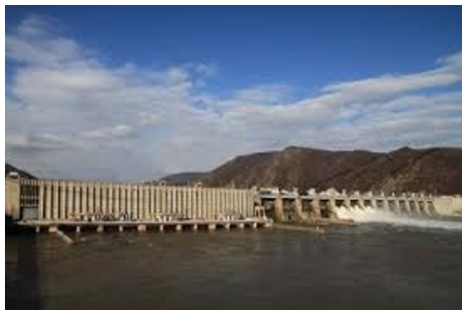
Fig. 1. Djerdap (Iron Gate) hydro plant Source: http://www.tos.org.rs/node/990
