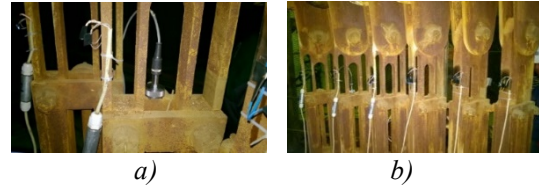
Figure 8: Measurements of acceleration (a) and deformations (b) on the cage connections tools
