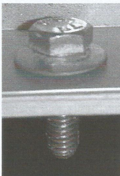
Fig. 9. The method of sealing the space between the screws and the structure
