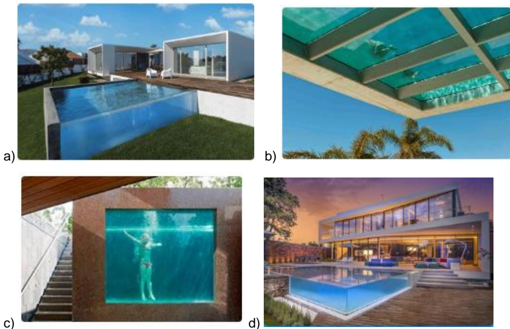
Figure 1. Acrylic pool window types: a) 3 side supported window; b) 4 side supported horizontal window; c) 4 side supported vertical window and d) L shaped vertical window
