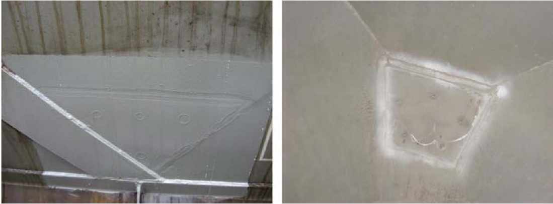
SI.6 Crack repair on the tanks
