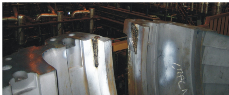
Figure 1. Example of detected and repaired cracked part of turbine housing
