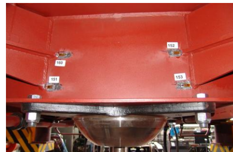
Fig. 5: Strain gauges 151 and 153
