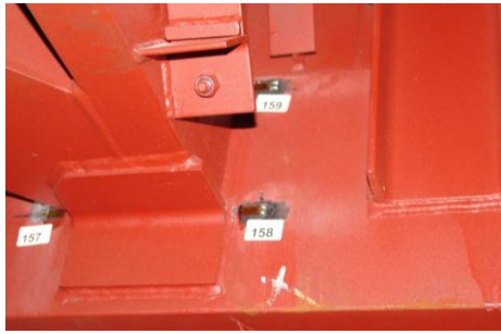
Fig. 3: Strain gauges 157, 158 and 159
