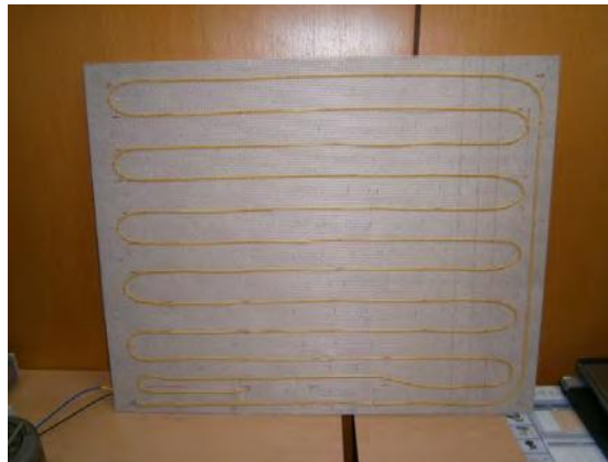
Figure 6. Detail of installation of the modify LTEFHP
