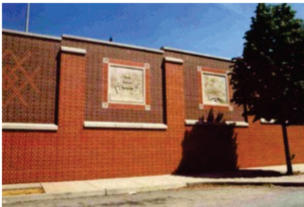
Figure 8. Panel inserts attached to a concrete barrier [1]
