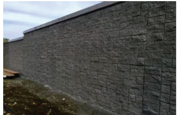
Figure 9. Sound barrier made of masonry blocks with broken stone edges [5]
