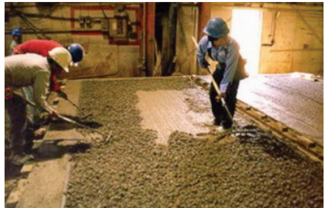
Figure 6. Final processing of the concrete barrier by raking [1]
