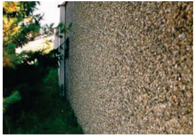
Figure 4. Concrete barrier with a surface in the form of a stone aggregate [1]
