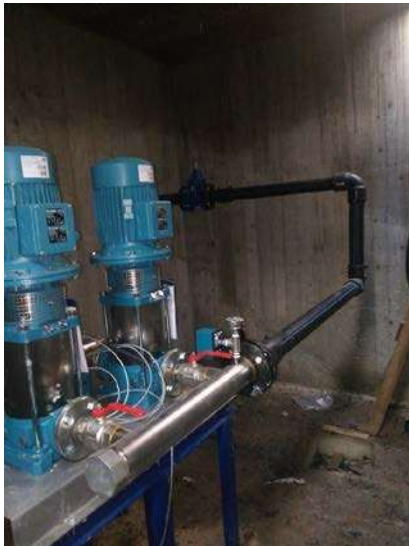
Figure 1: Interior of one water network manhole from city of Kraljevo
