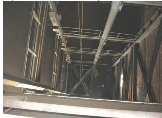
Fig. 5. Elevator embedment space - top view
