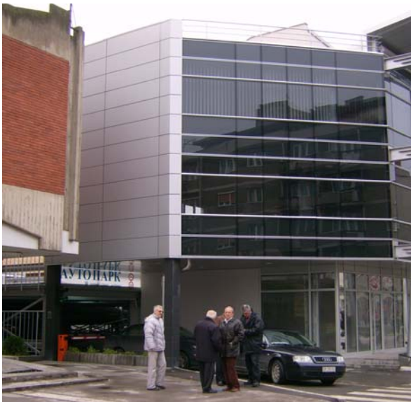
Fig. 13. Storey car park - Jagodina, capacity of 139 parking places
