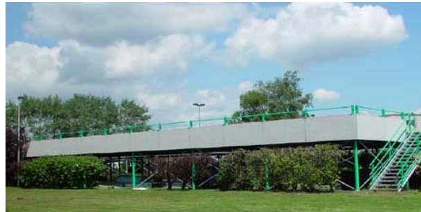
Fig. 5. Storey car park -Charleroi, capacity of 204 parking places
