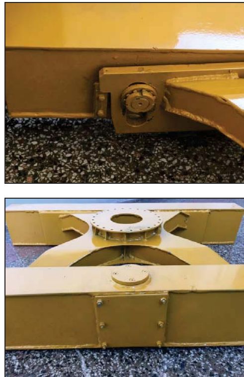
Figure 14. Central and auxiliary joints of the laboratory model of the joint connection [17]
