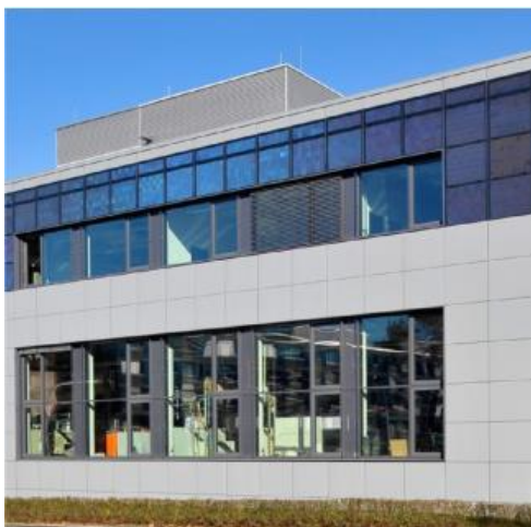
Figure 1. Rigid building integrated photovoltaic modules on a laboratory building of Fraunhofer ISE. The BIPV modules were developed and produced in a pilot production facility at the institute. © Fraunhofer ISE [4]
