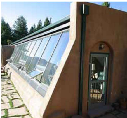
Figure 2 – Building designed with direct solar gains approach
