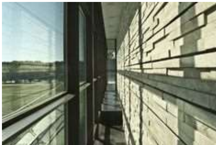
Figure 4 – Modern construction of the Trombe wall
