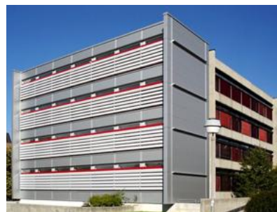
Figure 2 – Brise-Soleil usage on buildings
