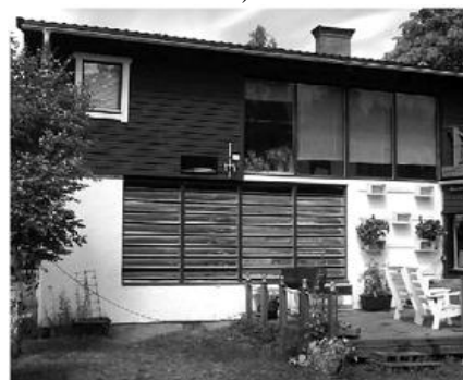
b) Figure 4 – Building-integrated multifunctional PV/T solar window, a) Solar window at Lund in the south of Sweden, b) The solar window in Solgarden, Sweden with closed reflectors
