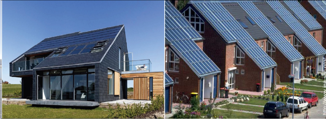
Fig. 4. Examples of Integration on Pitched roof
