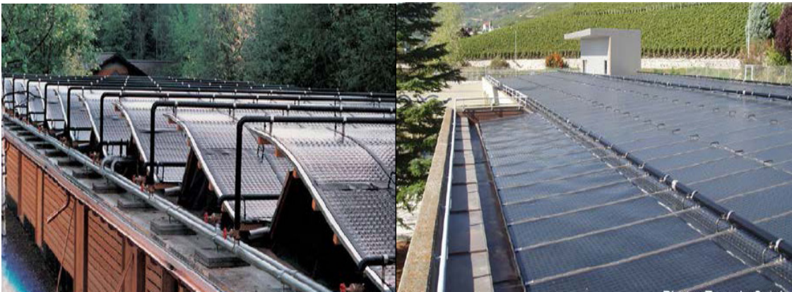
Fig. 5. Examples of Integration on flat roof
