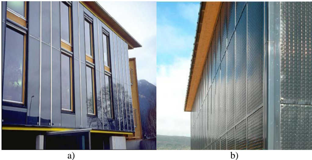
Fig. 2. a) Facade integration of glazed flat-plate collector, office building of AKS DOMA Solartedhnik b) Facade integration of unglazed flat-plate collector, CeRN, Switzerland
