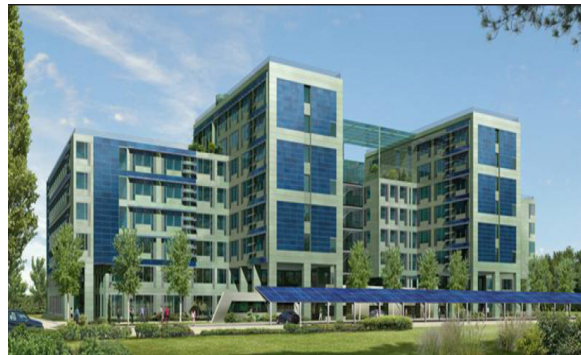
Fig.6 The Green Office in Meudon
