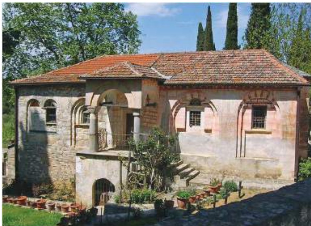
FIG. 1. Cemetery church of Chilandar Monastery. View from south-east, after: Kovačević 2016, 465, pic. 668
