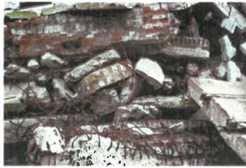
Fig.1 Typical construction waste ( www.hawersrecycling.co.uk )
