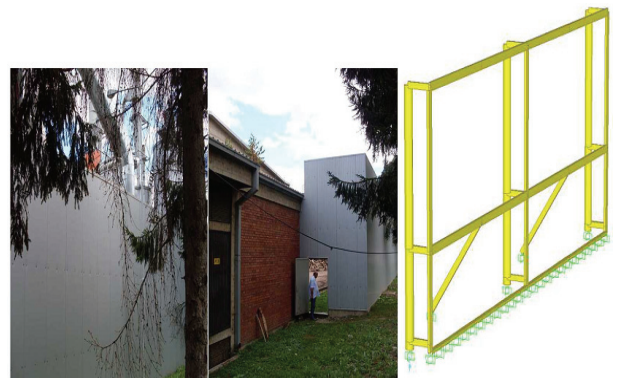
Fig. 5 Barrier and its base construction
