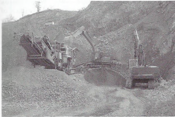
Fig. 5 Set of the construction mechanization necessary for operations in the quarry
