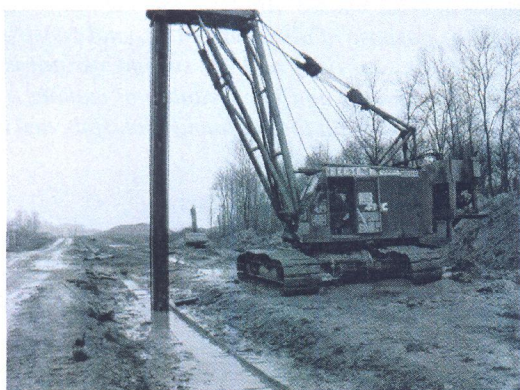
Figure 2: Excavation of the diaphragm trench
