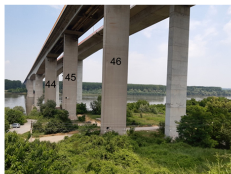
Figure 8. Bridge on the Beška landslide.
