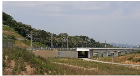
Figure 7. Viaduct on the Čortanovci landslide zone of the Sloboda bridge.
