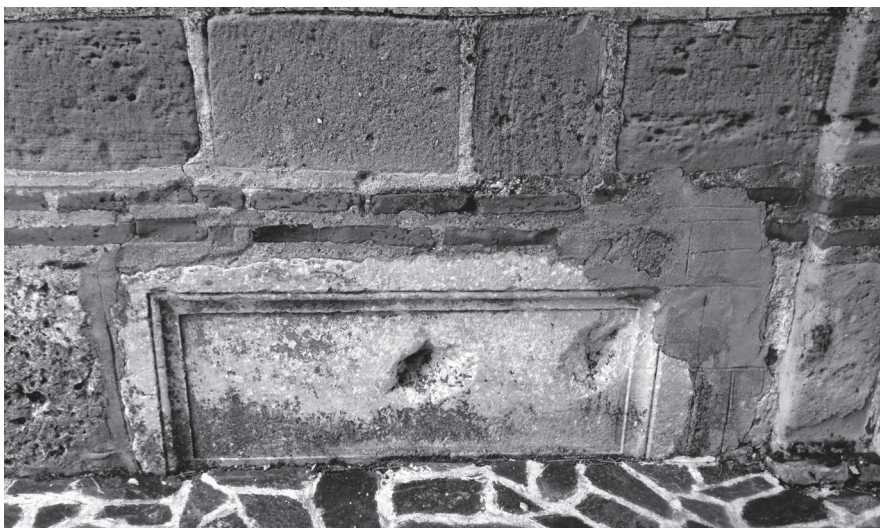
Fig.4. Spolia inserted at the lower register of the north wall, St. Nicholas Church, Ljuboten, photo: Jasmina S. Ćirić
