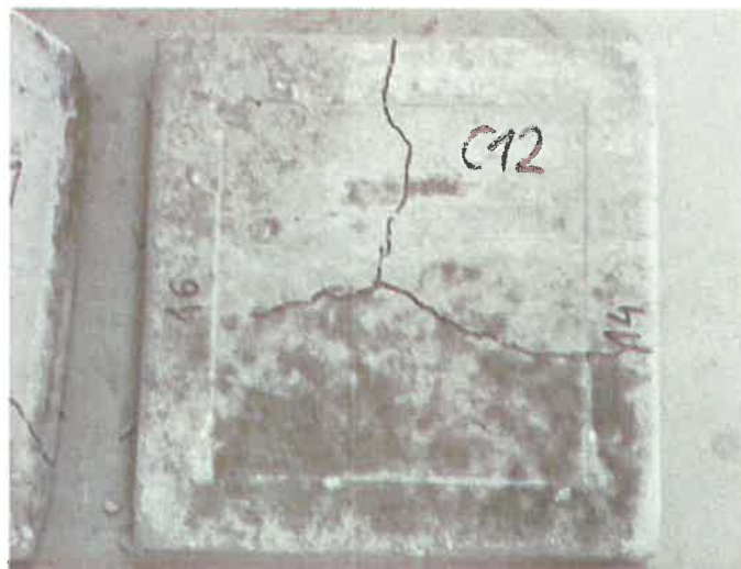
Figure 4. Concrete slab specimen after impact resistance testing
