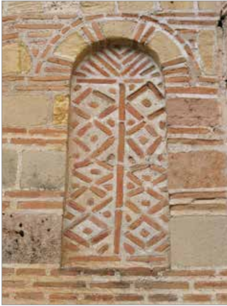
Fig. 4: Niche with rhombus brick ornamentation, the apse of St. Demetrios Church, Mark's Monastery, photo: © Jasmina S. Ćirić
