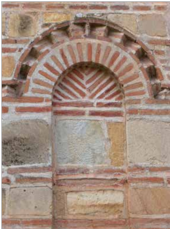
Fig. 7: Tree of Life brick ornament of the apse of St. Demetrios Church, Mark's Monastery, photo: © Jasmina S. Ćirić
