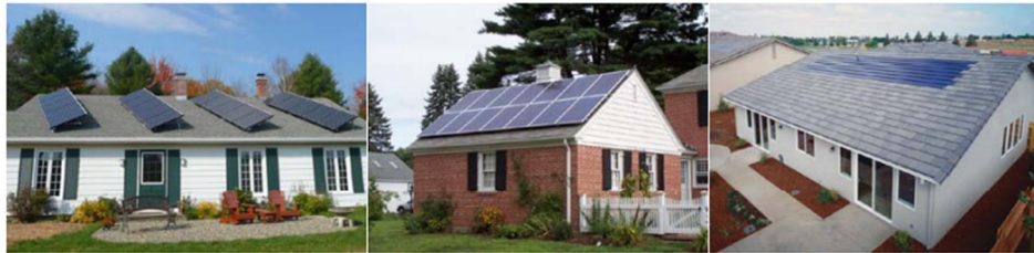
Figure 3: Examples of increasing integration of PV Panels [14]
