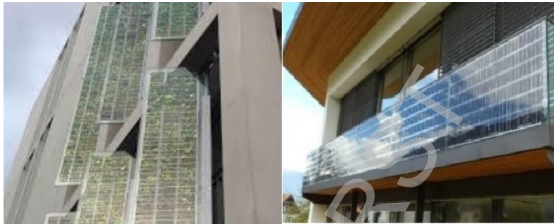
Figure 8: BIPV systems on external integrated devices [20]
