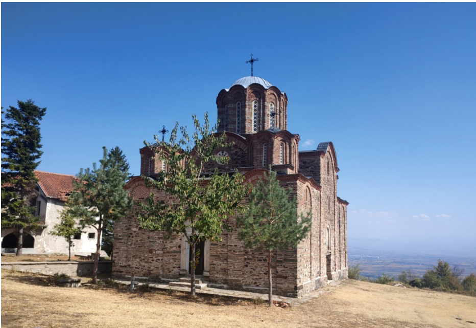
Figure 4. General view of the church exterior, seen from the southwest (Photo: Jasmina S. Ćirić)
