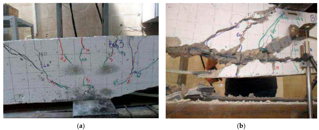
Figure 32. Experimental G3 beam failure: (a) mid-support section; (b) mid-span section.
